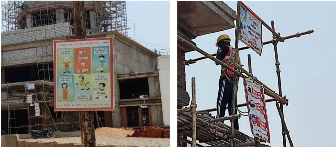
Figure 26: A good Example of Safety signage displayed on site.
