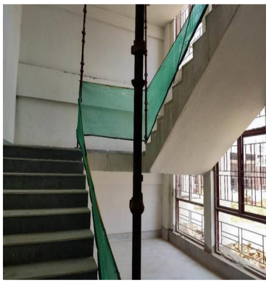
Figure 25: A good Example of Safety nets and barricading to be provided on site.
