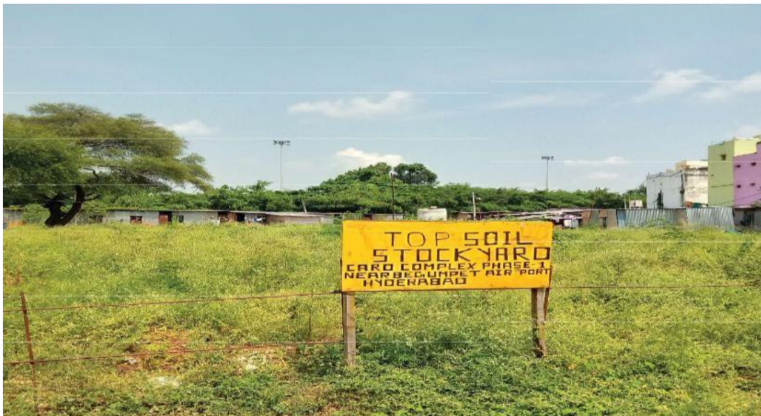
Figure 11: A good example of top soil preservation on a site.
