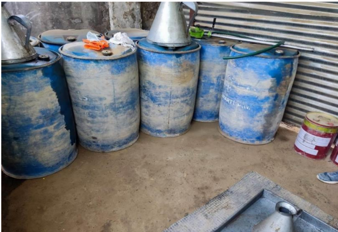
Figure 9: A good example of hazardous chemical drums stored on an impervious surface in an enclosed area on site.
