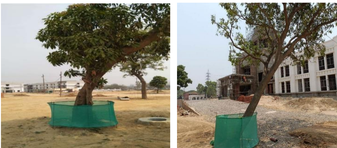
Figure 10: Good examples of barricading existing trees on site.
