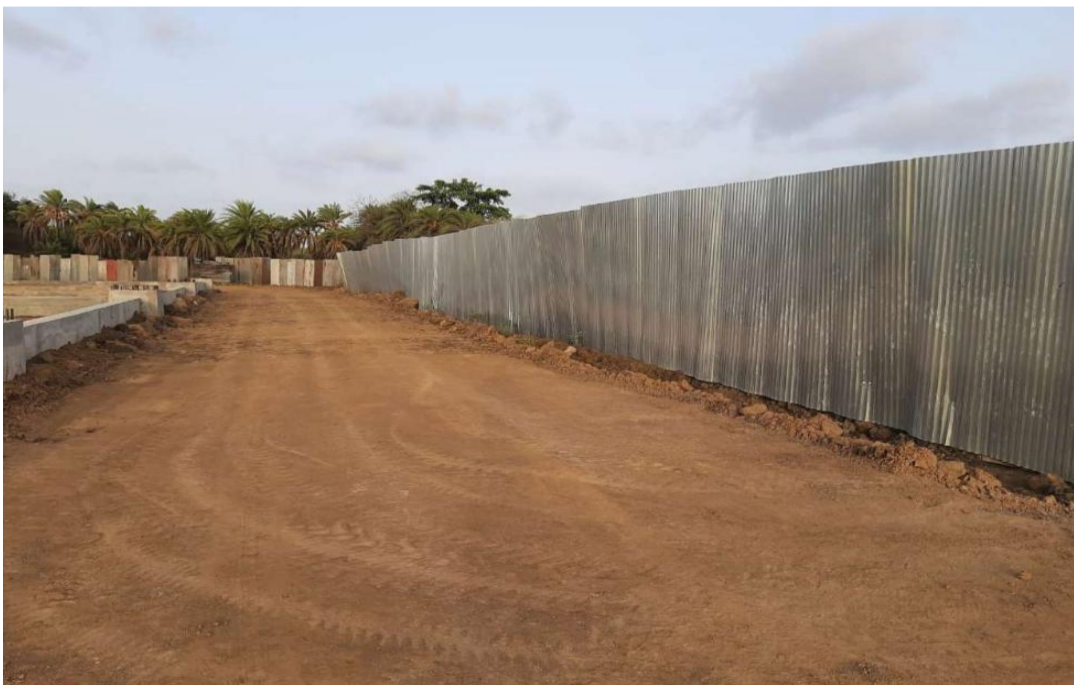
Figure 4: A good example of 3-meter-high barricading using GI Sheets
